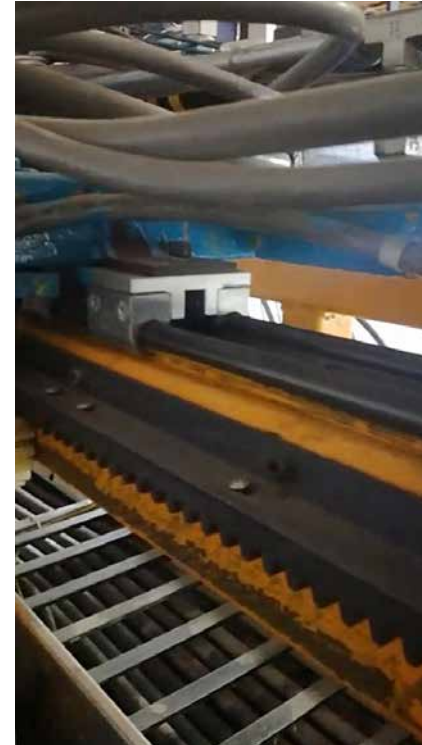
Refrigeracion Ojeda, Luis Garcia Maceda, Mexico City, Mexico
